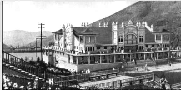
Columbia Gardens pavilion, from an old post card.
