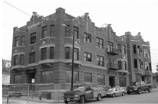
SAVED: The O'Rourke (Quartz at Alaska Street; see also page 124) was saved by volunteers who paid back taxes and commissioned a structural analysis of the building. Photo courtesy Butte CPR.
